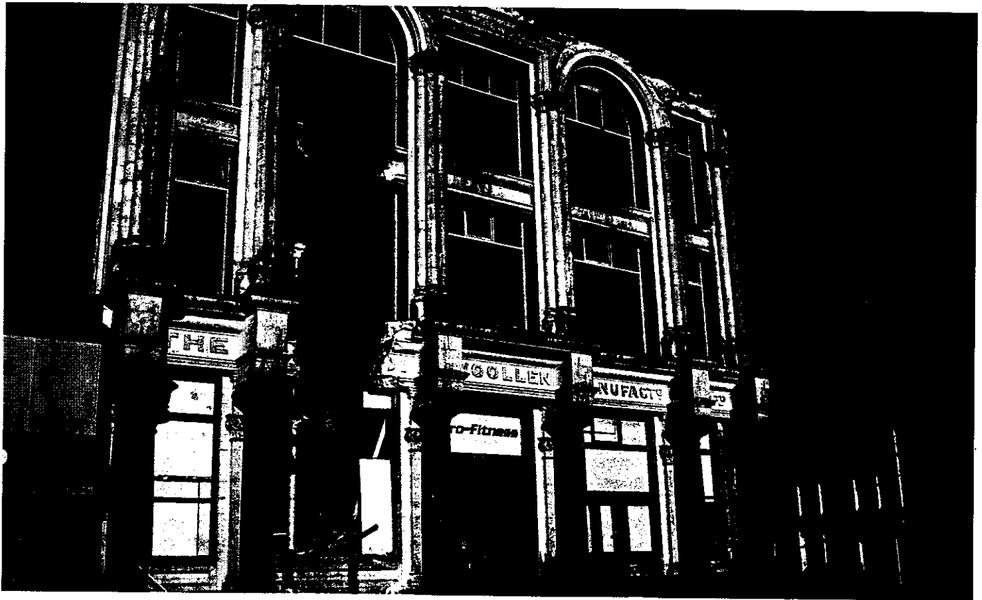
Above: The now demolished Kiapoi Woollen Mill.
