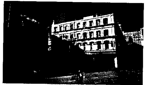
Top: Dunedin Railway Station – now converted to a Valentines Restaurant.
