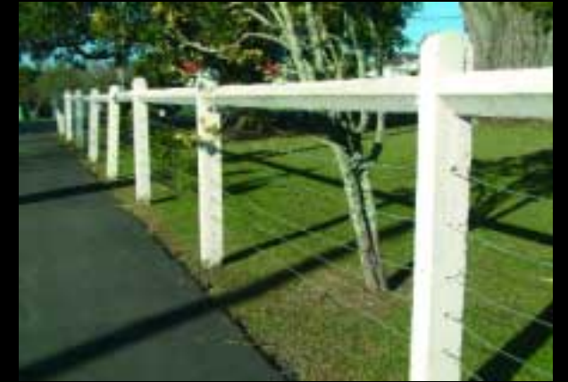
Post and wire fence
