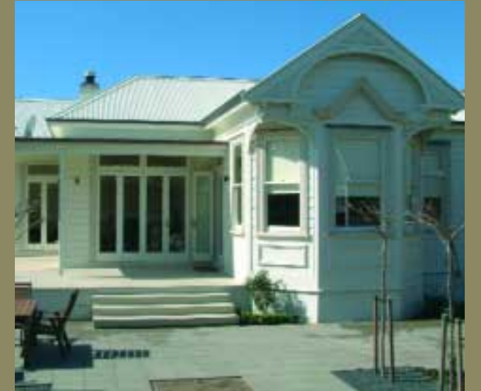
A gable bay addition identical to the existing bays was used to extend this house.
