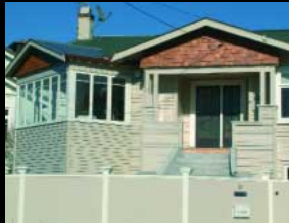
Bay windows are a good way of allowing light in and providing extra space in rooms where any greater change will affect the character of the house.
