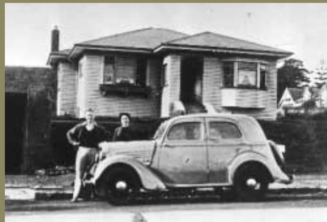
House in Lake Rd, Belmont, 1940s. Takapuna Library.
