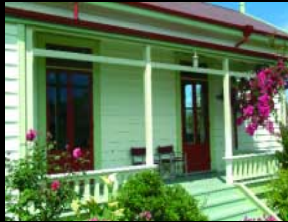
Consider installing French doors that are of a similar period or profile to other joinery.
