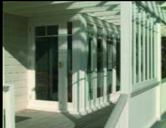
Use larger glazed openings at the rear of the house with proportions similar to those of existing windows or doors.
