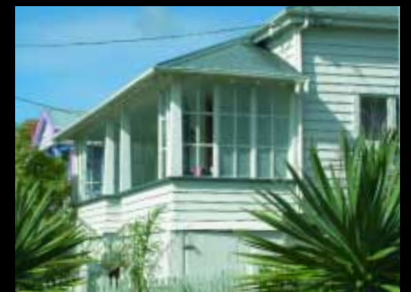
Replace later windows with glazed verandah panels common to the style of the building.
