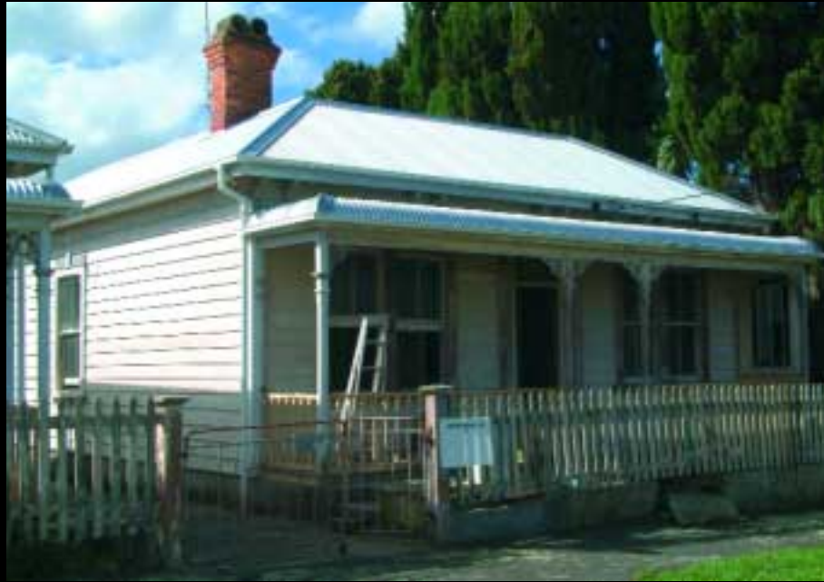
This roof was reclad keeping the existing form.
