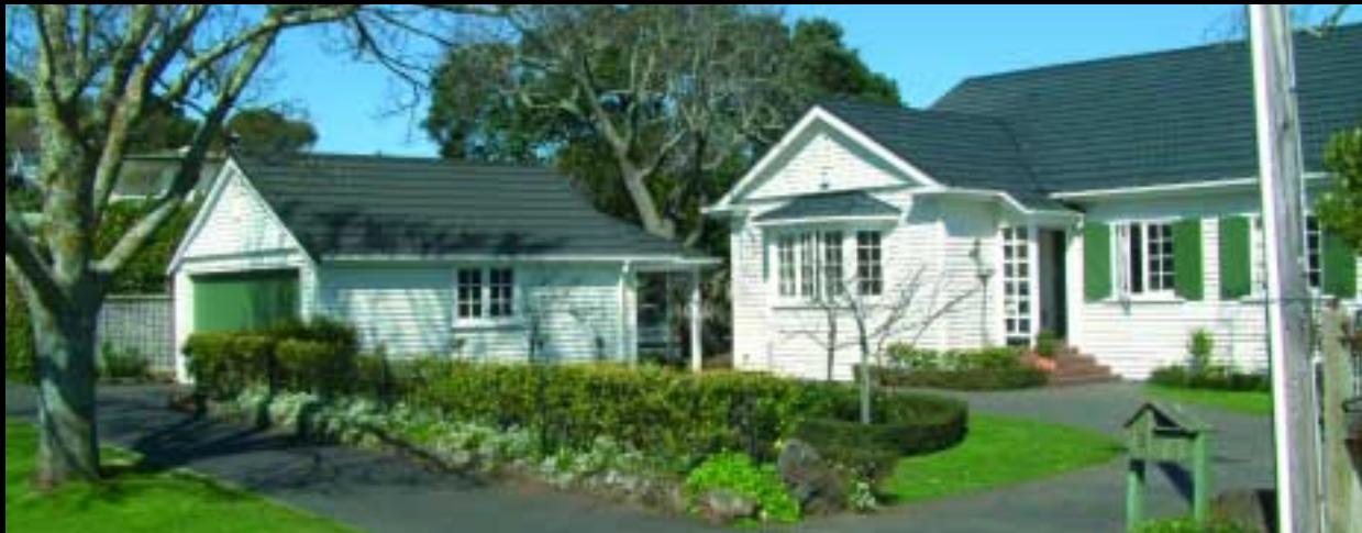
Keep the garage free-standing and use a complementary design to link it to the house.
