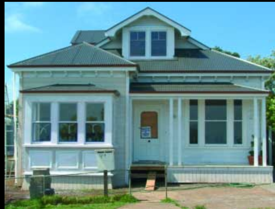
A new gable was added to the existing roof by building within the roof valley on this house.
