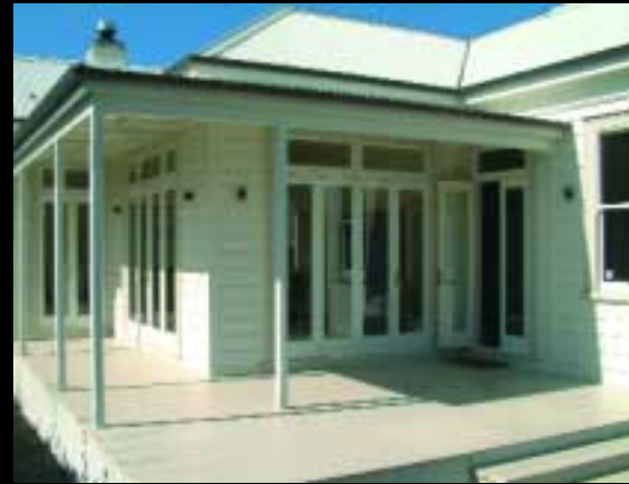
Reduce the visual impact of larger windows and doors by containing them under a verandah which will also provide shelter from bad weather.
