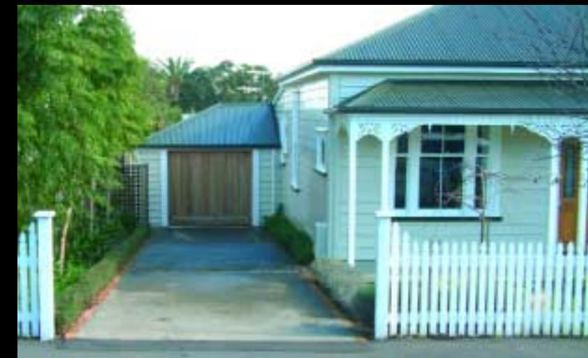
Where the garage is in a side yard consider whether it needs to be attached to the house or separate. If attached, make sure the front of the garage is at least 600mm back from the front of the house.
