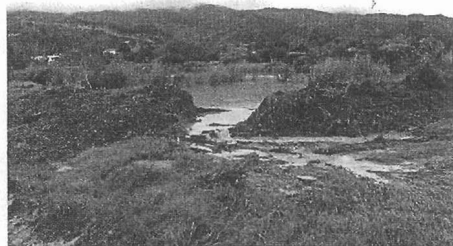
Figure 5 (right): The dyke that failed to keep floodwaters out of the retirement village at Coromandel. Furniture and vegetation debris suspended at the top of the fence line shows how high the floodwaters were with respect to the dyke. The remainder of the floodplain that was well submerged during the event is visible to the left.
