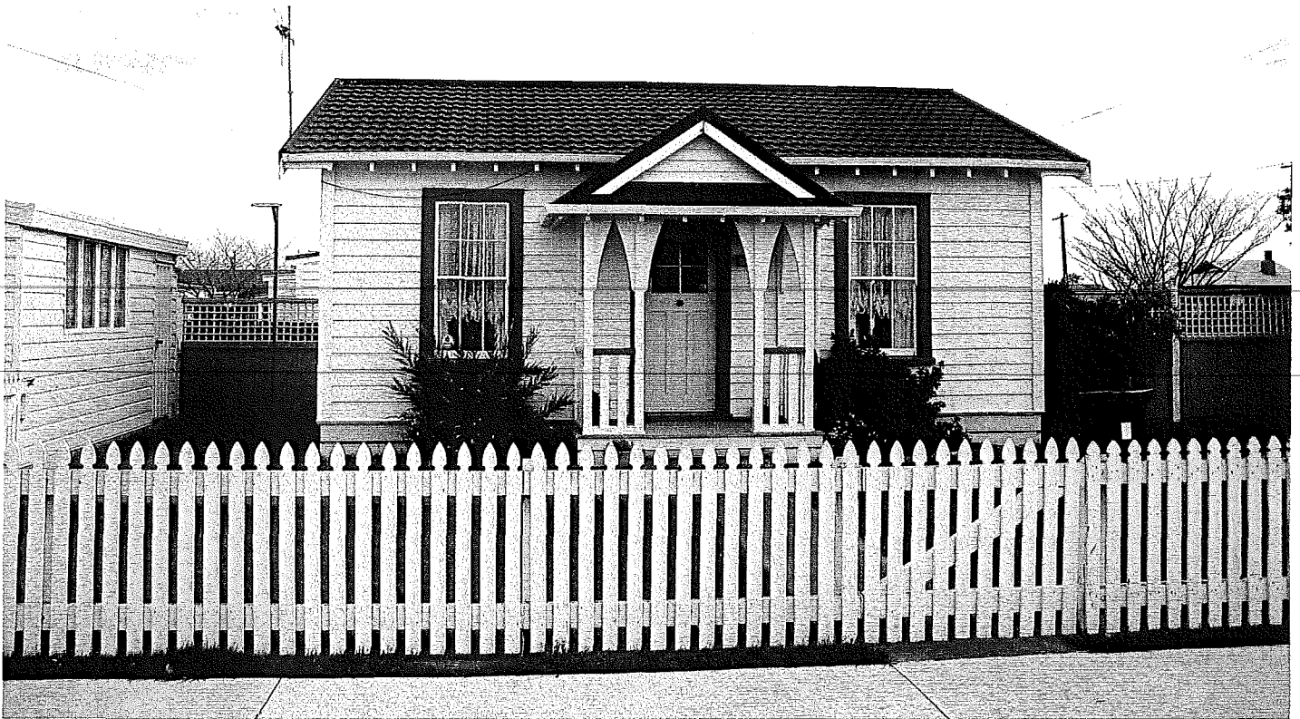
ABOVE: A restored AB 296 Roof A porch A cottage from Milson. A tile roof has replaced the original iron and the chimney has gone but original windows and doors remain. Of the four basic AB 296 designs this particular style seems to hold particular appeal to home restorers perhaps because of its 'cottage like' look. The paling fence in front of this property was another distinctive feature of the Milson sections.
