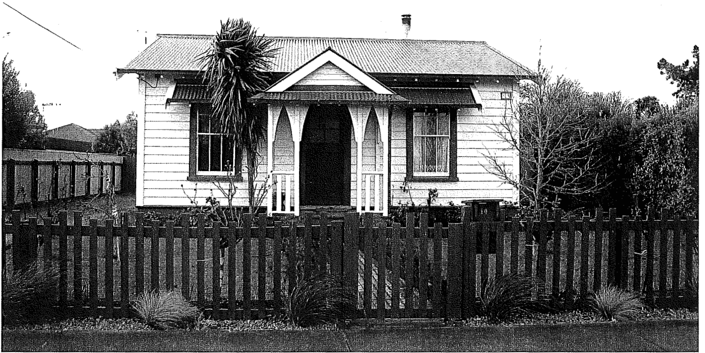
ABOVE: Renovated AB 296 Roof A Porch A cottage at Milson in Palmerston North. Small rectangular plaque on the top right hand side under the eaves displays the factory number. Only two of the Milson houses appear to retain these numbers which provide another means of dating the house. Originally Milson railways staff had mail delivered on the basis of house numbers, but because sequentially numbered houses were not side by side this caused difficulties until residents petitioned Railways to be allowed to display more conventional street numbers, which was granted as long as they were only on the gates and not the houses.
