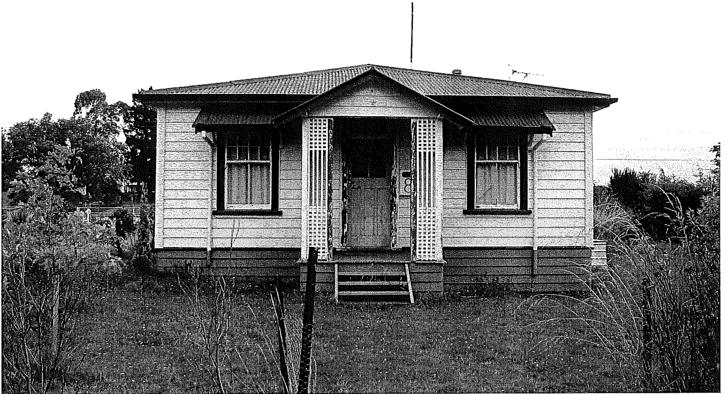
ABOVE:: Railway house from the Frankton factory situated at Ohakune; it is of the AB 296 type with Roof A and probably a subsequently modified porch A. Some of the Ohakune houses have enjoyed a new lease of life as ski season chalets.
