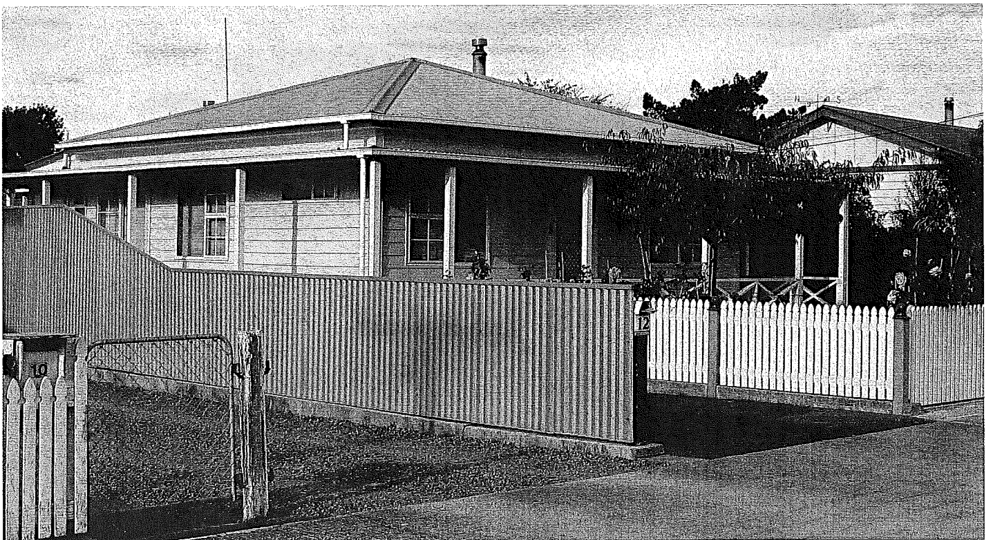
ABOVE:: Much modified AB 296 Roof C Porch C Frankton railway house. This example has had the original porch replaced by a wraparound veranda and new window frames.
