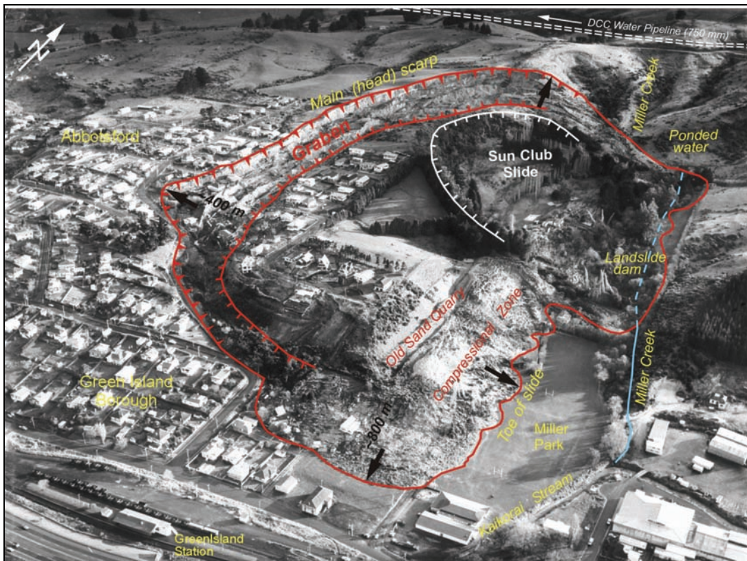
Figure 3.3 Oblique aerial photo of the Abbotsford Landslide taken on 9 August 1979, the morning after the final movement occurred. The landslide mass moved c. 50 m down a 7° bedding plane clay layer in about 50 minutes, forming a graben 70-150 m wide at the head. Features seen here that contributed to the landslide include the old sand quarry at the bottom of slope (which was closed in 1969), and a leaking water main c. 200 m north (up slope) of the landslide. The old Sun Club Slide on the west side of Miller Creek (dammed by the landslide) shows the inherent instability of the area. (Photo by courtesy of Aeropix, Dunedin)
