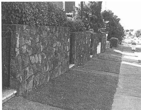
Above: A physical barrier
